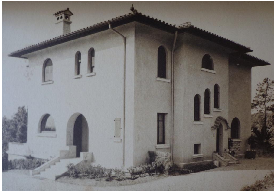
FIG. 01: Villa "Les Bougainvillées", Var.
